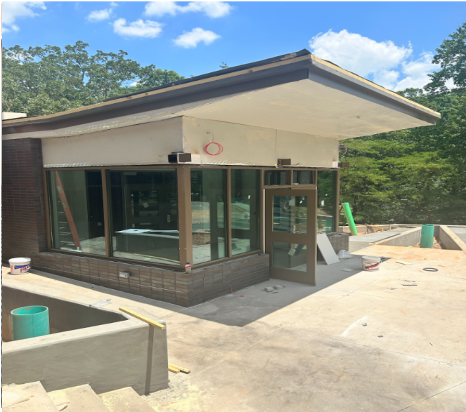
Entry vestibule storefront installed
